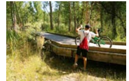
BICYCLISTS HAVE DIFFICULTY ACCESSING SOME TRAIL SEGMENTS
