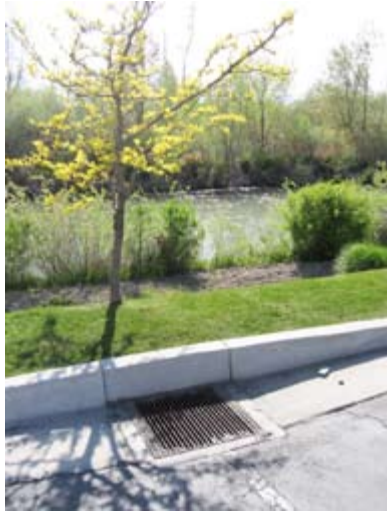
WATER RUNNING OVER IMPERVIOUS SURFACES COLLECTS POLLUTANTS AND DRAINS INTO THE JORDAN RIVER
