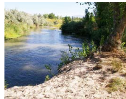
ERODING BANK ALONG THE RIVER
